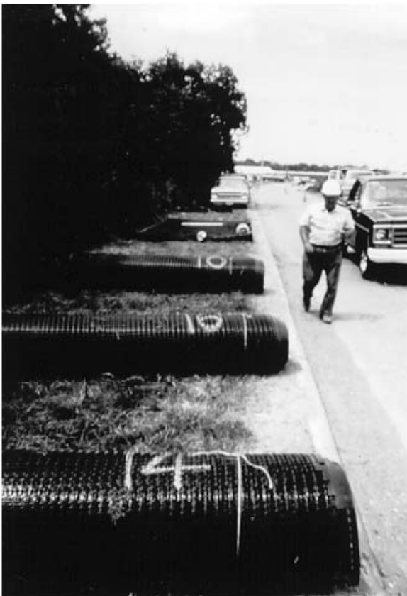
Figure 11-2. Inspect reinforcing elements: top photo shows a variety of reinforcements including metallic strips, welded wire mesh, and geosynthetics and bottom photo shows reinforcement length painted on geogrid reinforcement.
