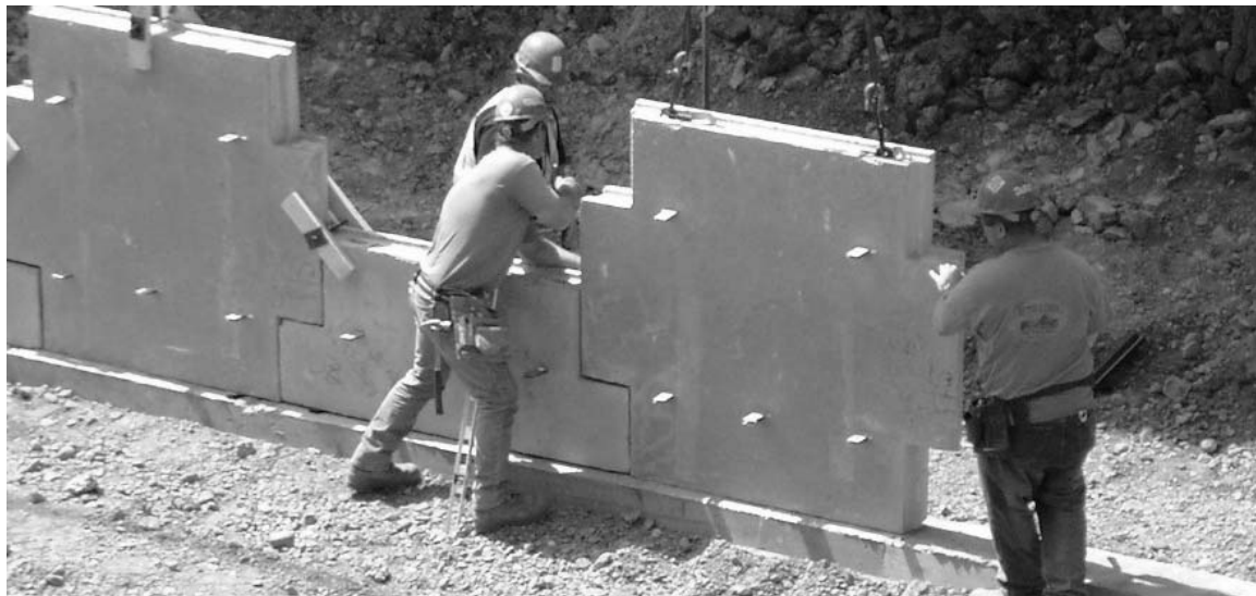
Figure 11-3. Concrete leveling pad showing: a) leveling the concrete, b) completed pad, and c) placing the facing elements on the leveling pad.
