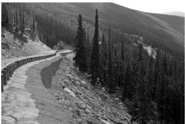
Figure 2-22. Guanella Pass wire-faced wall.
