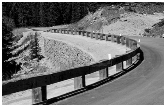
Figure 2-23. Guanella Pass architectural concrete faced wall.
