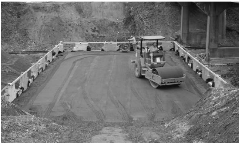
Figure 2-10. Compaction of the reinforced wall fill.
