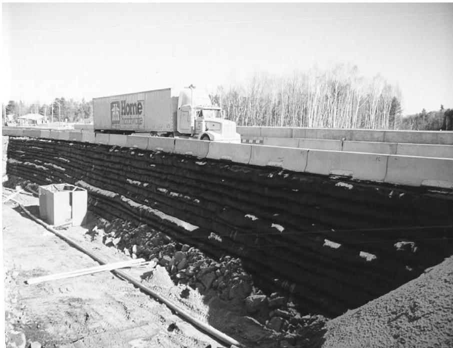
Figure 2-3. MSE wall used to temporarily support a permanent roadway embankment for phased construction.
