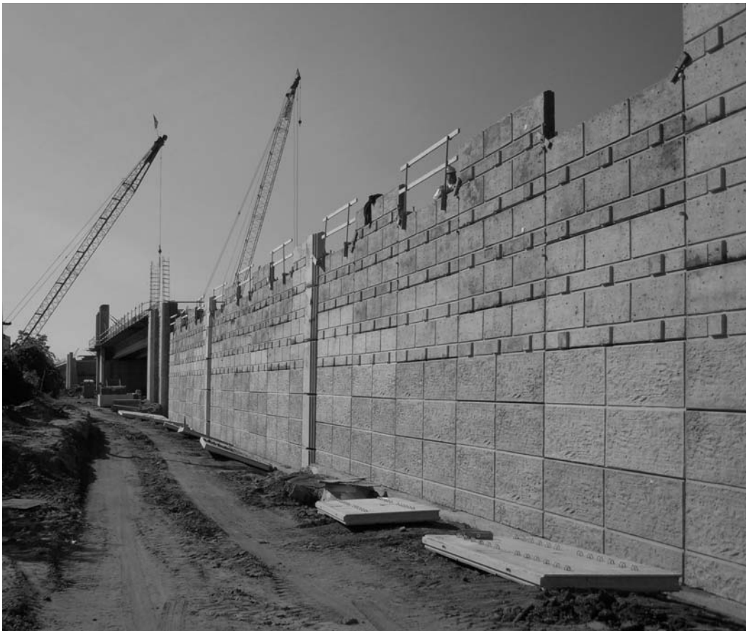
Figure 2-17. MSE wall construction on Mn/DOT Crosstown Project, 2008.
