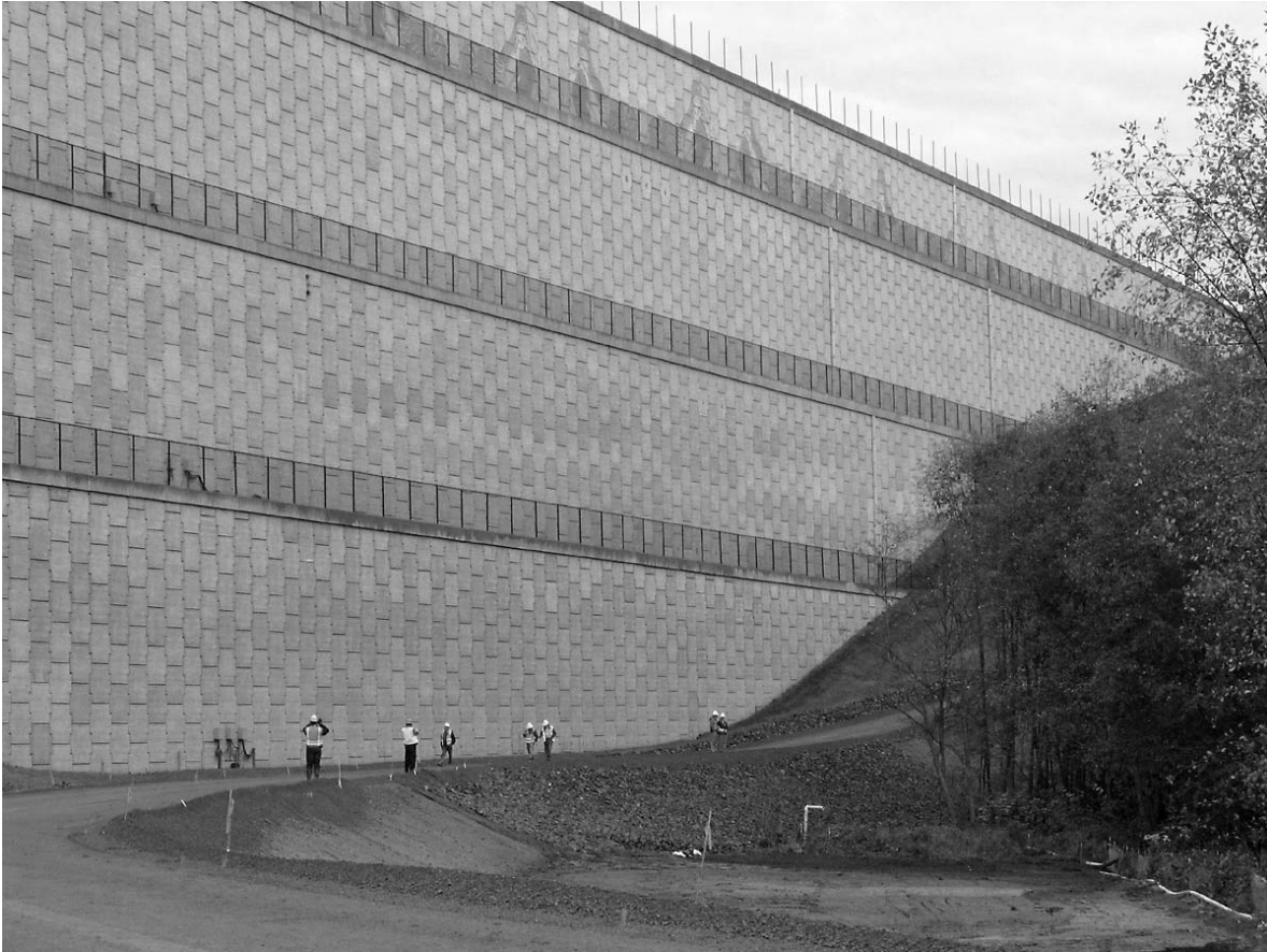
Figure 2-21. SeaTac Airport runway extension MSE wall.
