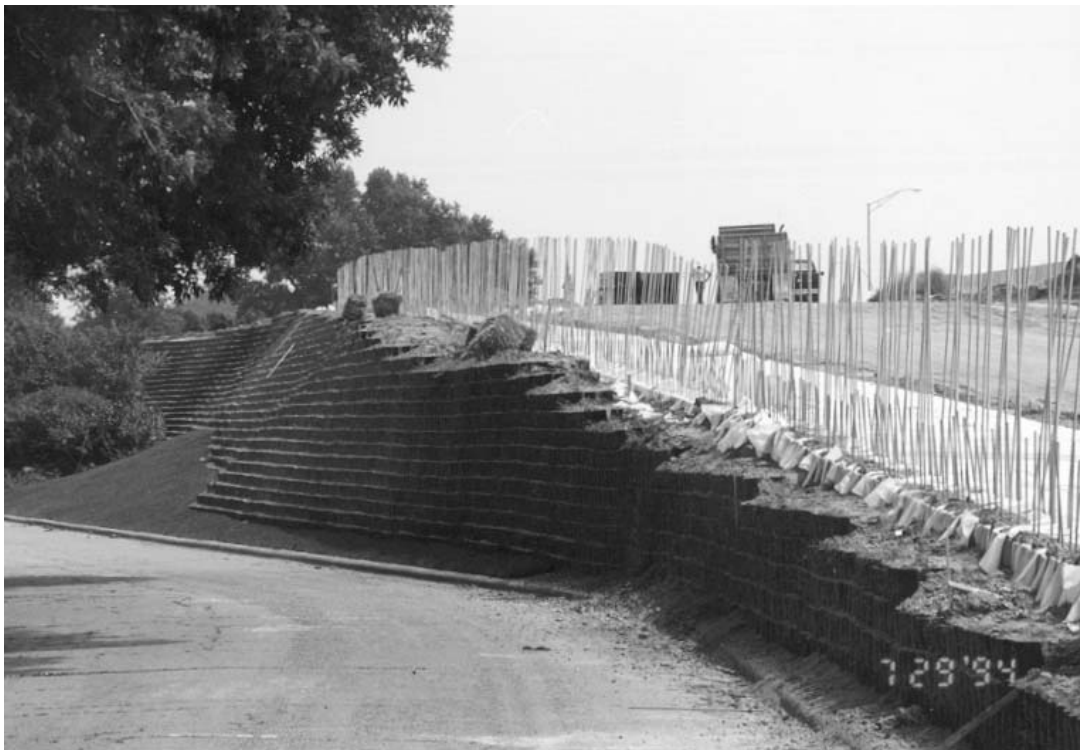
Figure 3-9. Geocell face unit with vegetation.
