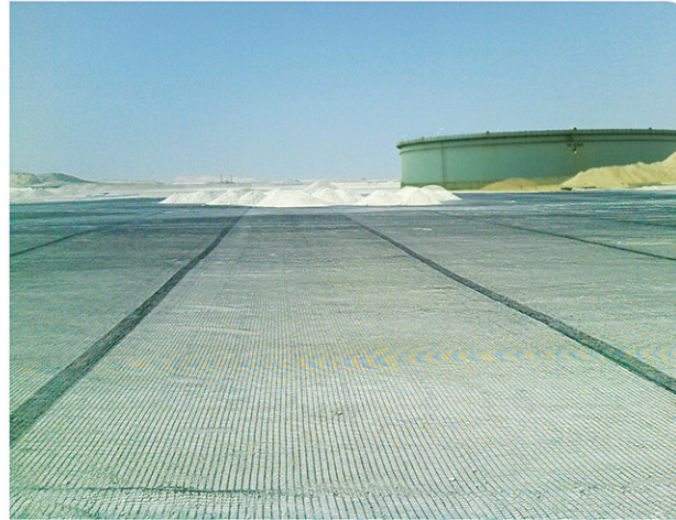
■ soil stabilization - United Arab Emirates
