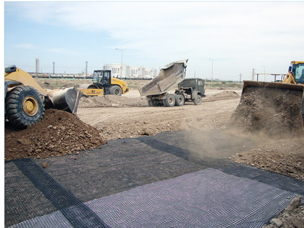
■ soil stabilization in Baku-Azarbaijan
