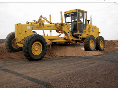
■ Sub-soil reinforcement with GPGrid2BX_Geogrid, Qom-Garmsar new Railways
