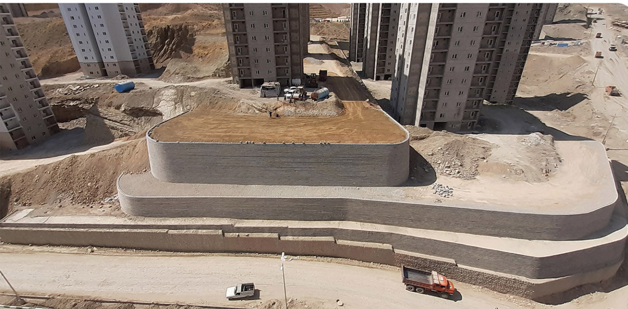
■ Geogrid reinforced retaining wall, Pardis new town
