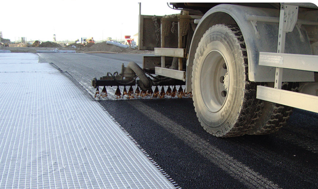
■ Asphalt overlay implementation, Baku Azerbaijan
