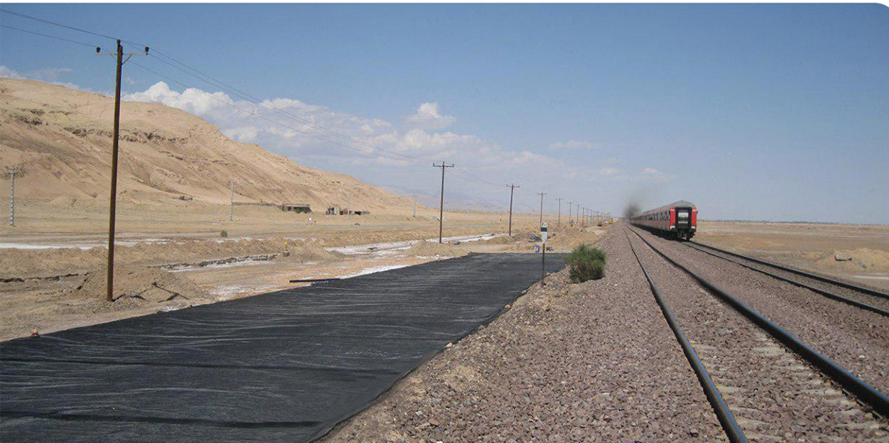
■ Sub-soil reinforcement with GPGrid2BX_Geogrid, Qom-Garmsar new Railways
