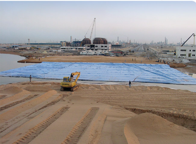
■ soil stabilization in khor Jafari
