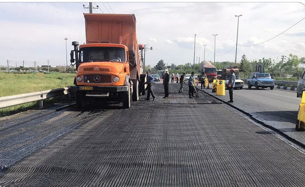
■ Asphalt overlay reinforcement, Karaj
